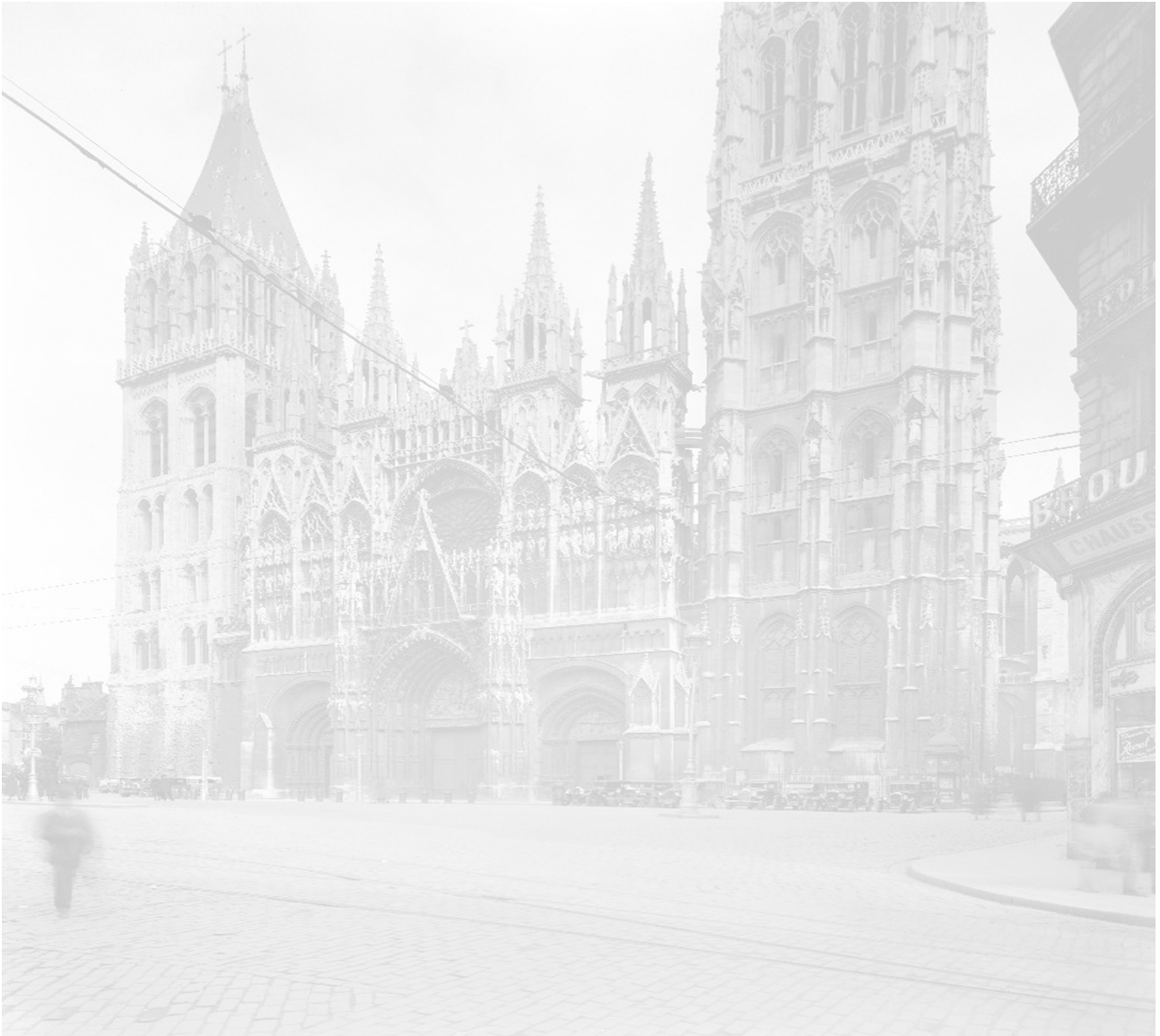
West façade of Rouen Cathedral Clarence Ward Archive Department of Image Collections National Gallery of Art, Library, Washington, DC
